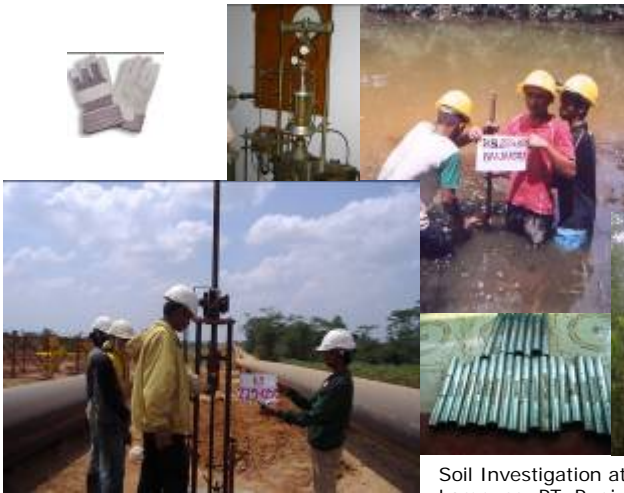
Soil Investigation at Lampung, PT. JFE Engineering Corp
