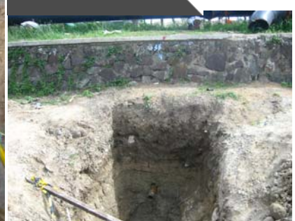
Pilot pipe at target shaft
