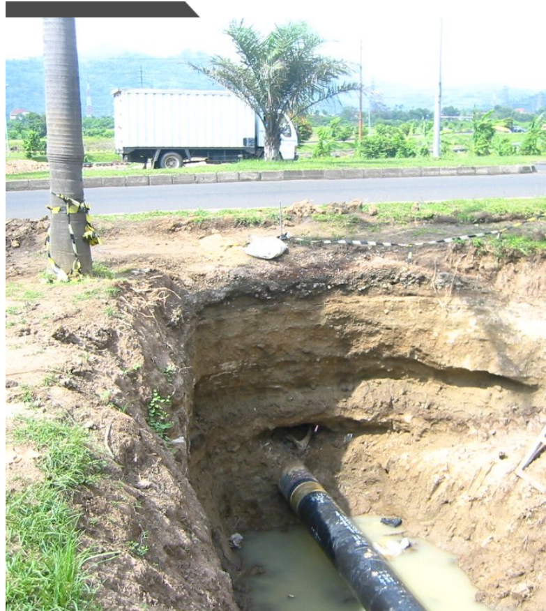
Completion of Works
