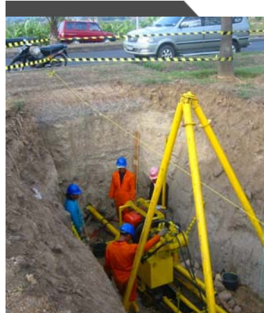
16" thrust boring at Cilegon – Banten
